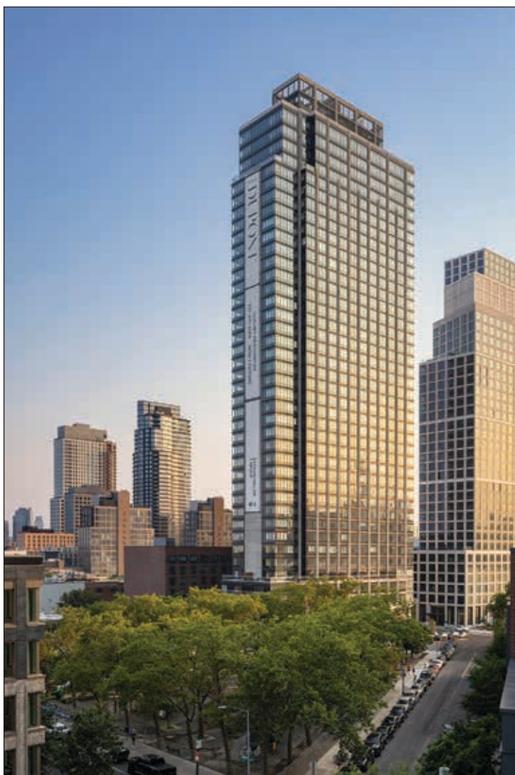
The Dupont, Rockefeller Group’s new residential rental tower near the waterfront in Greenpoint, Brooklyn
